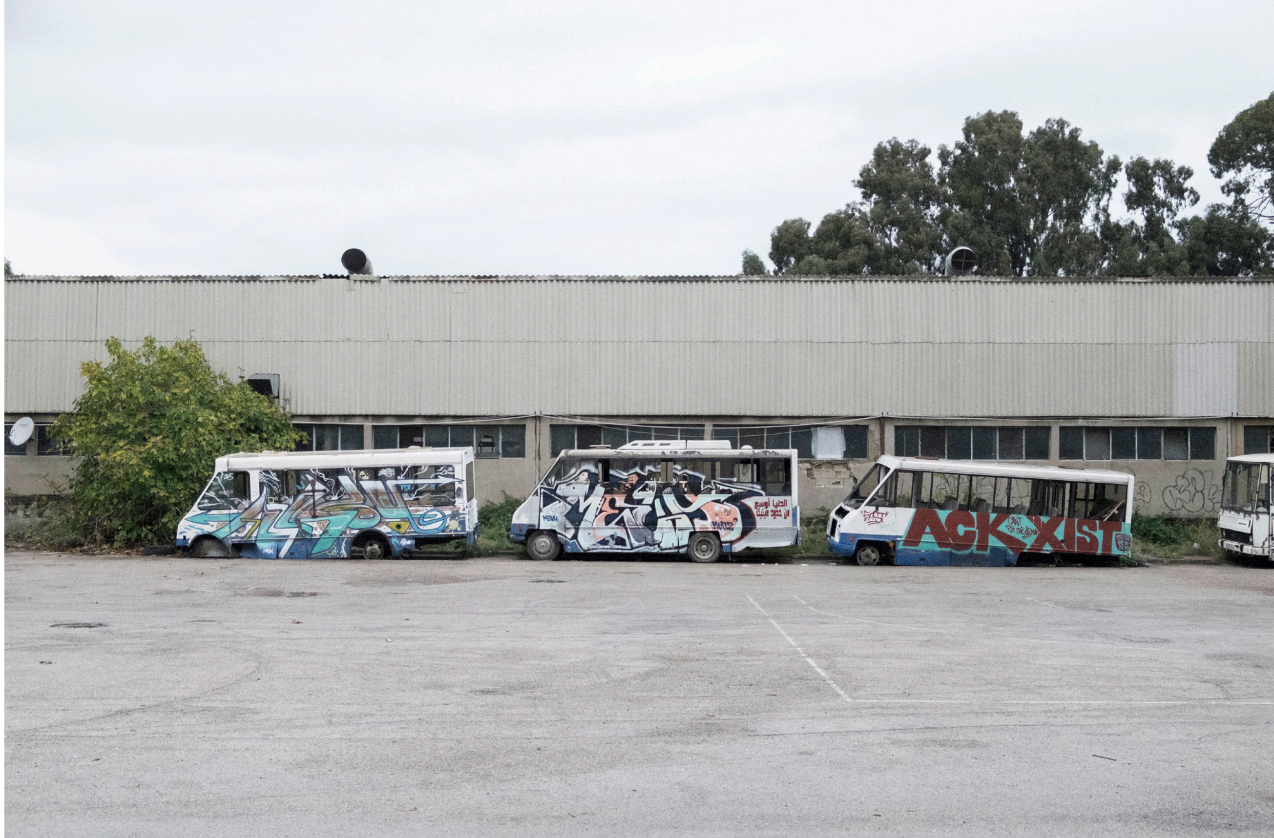
Hangar for bus park
