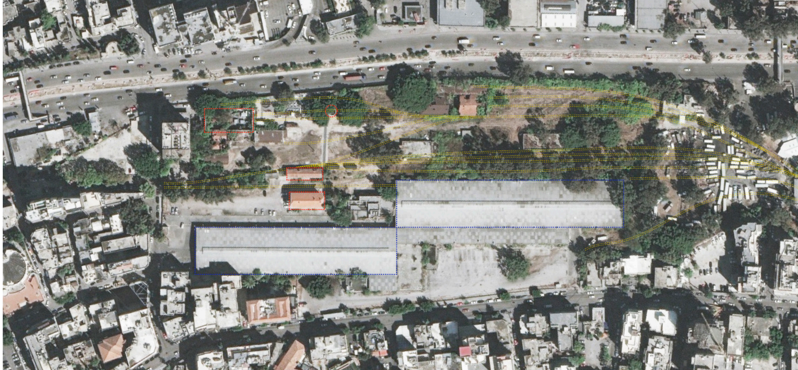
Rail tracks Hangar for bus park Train station built heritage
