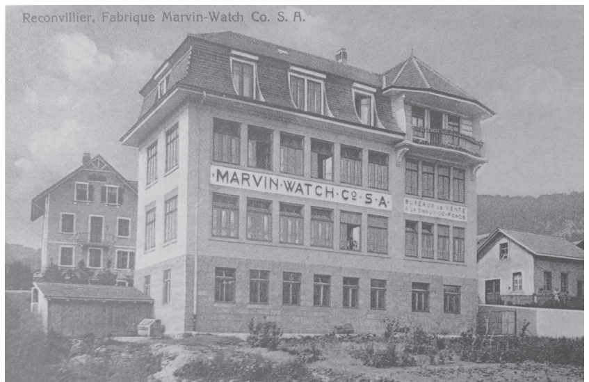
Fig. 37 Factory building, photo undated (Histoire de Reconvillier, 1984)
