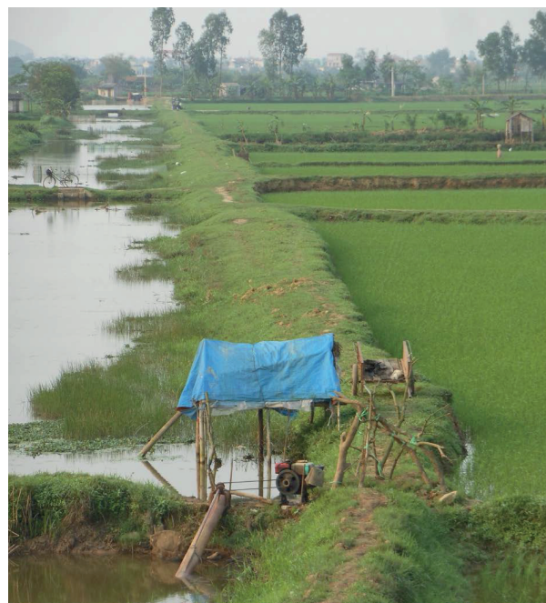
Figure 30 Station de pompage portative, Ninh Binh
