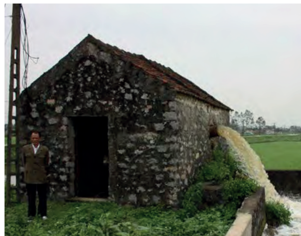
Figure 29 Station de pompage, irrigation, Den To
