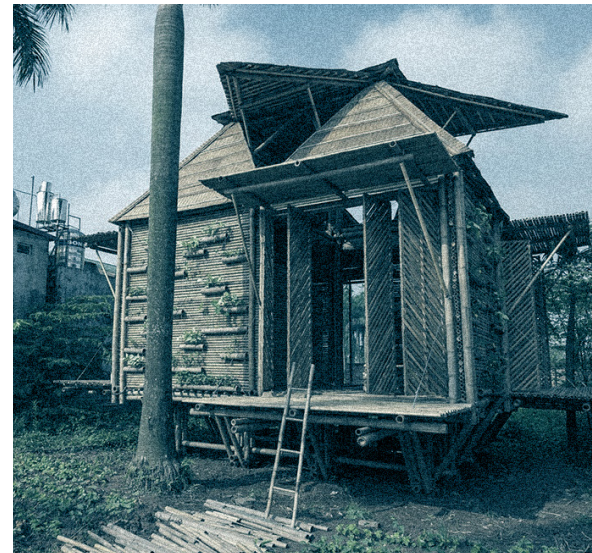
Blooming Bamboo House Cau Dlen Town, Ha Noi, Vietnam 2013 H&P Architects
