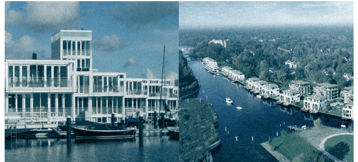
Floating Houses Village Amsterdam, Pays-Bas 2011 Architectenbureau Marlies Rohmer
