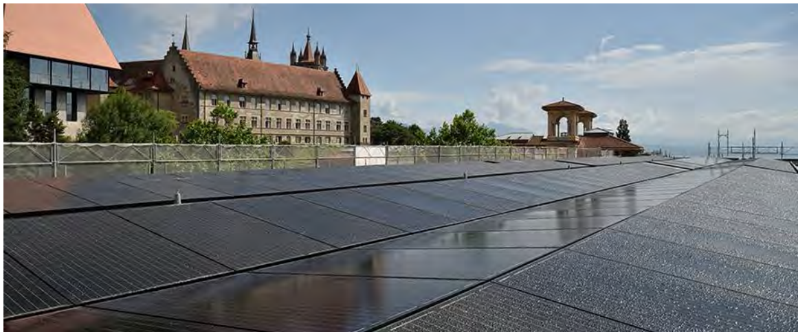
Figure 10. View of the photovoltaic roofing.
