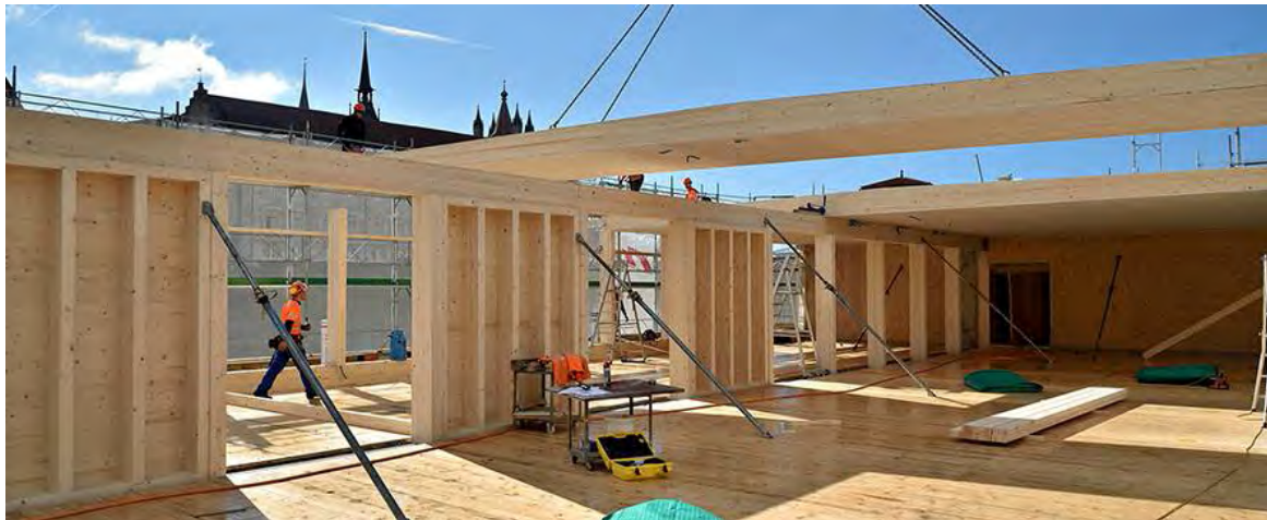
Figure 8. On-site assembly of the prefabricated wooden elements.
