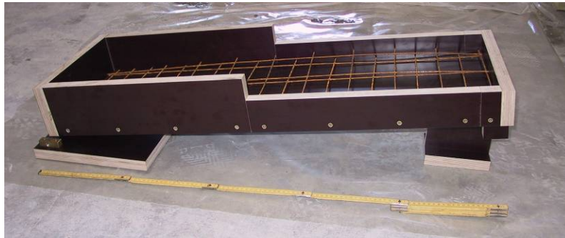
Figure 4-2: Test set-up for the sensitivity to a slope
