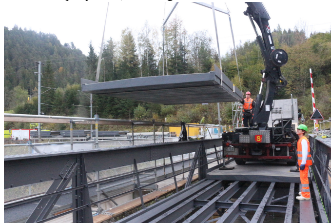
Fig. 3: Assembly of a sandwich slab element.
