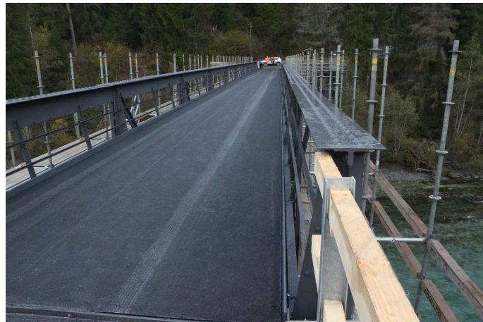
Fig. 1: Asphalted GFRP-Wood slab with steel guard rails.
