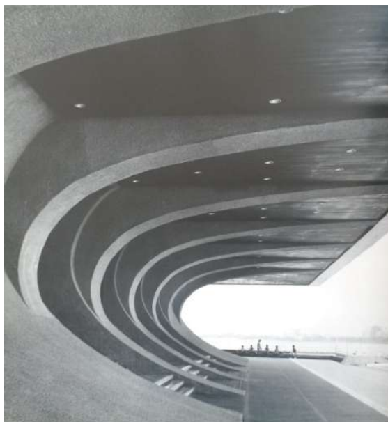
Leandro Locsin_Theater of Performing Arts_(1967)_Pasay Vue du portique Source: POLITES (1977, photo Akio Kawasumi)
