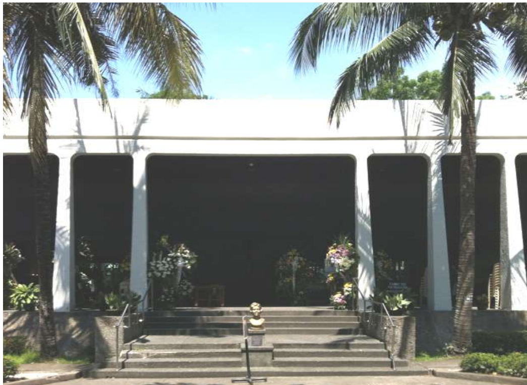
Leandro Locsin_ de la Salle Chapel (1956)_Bacolod City, Negros occidental Entrée principale Source: google earth
