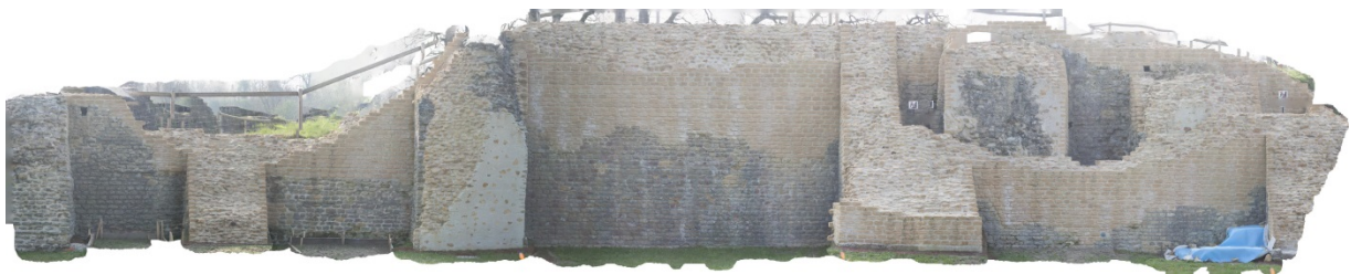
Figure 8: Restoration of the masonry of the north wall (orthoimages)
