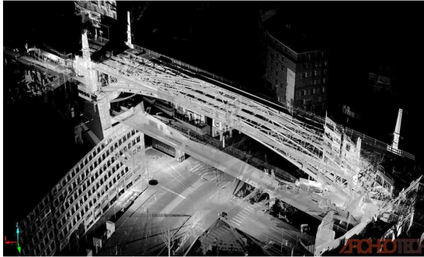
Figure 1: 3D scan of the Bessières Bridge in Lausanne ( Archeotech )
