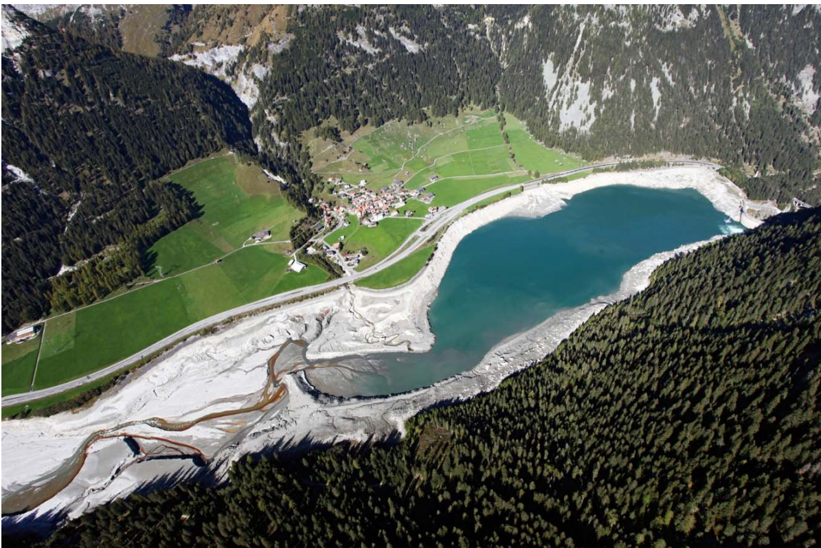
Figure 1.1: Sedimentation of Sufers Reservoir located in Grisons, Switzerland (photo courtesy of Kraftwerke Hinterrhein AG).
