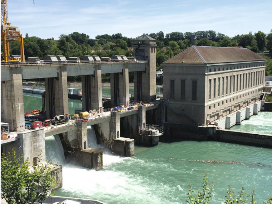
Fig. 1 Picture of the Chancy-Pougny run-of-river dam, location on the Rhône River, on the border between Switzerland and France (i.e. dam with the 4 spillway gates on the foreground, power plant on the background)
