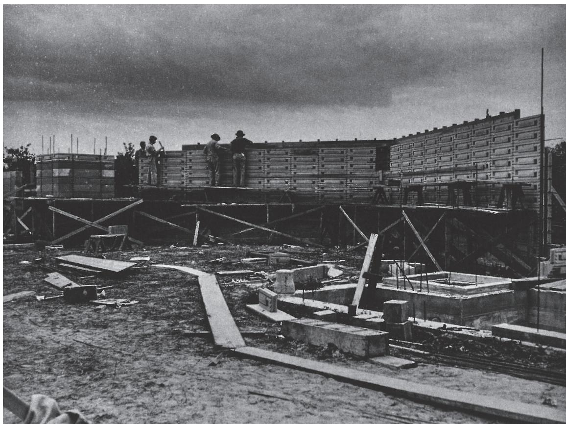
[fig.8\_Florida Southern College construction, Lakeland (1938)] This photo shows a team of student laborers building the lower cast block walls of the Pfeiffer Chapel. FLLW 3816.045
