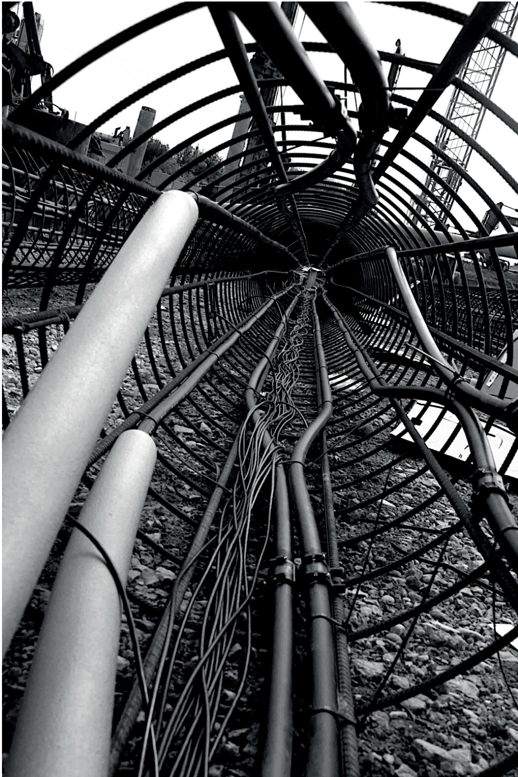
Figure 1.12: Typical pipes and thermal insulation in an energy pile (image courtesy of Dr. Thomas Mimouni).
