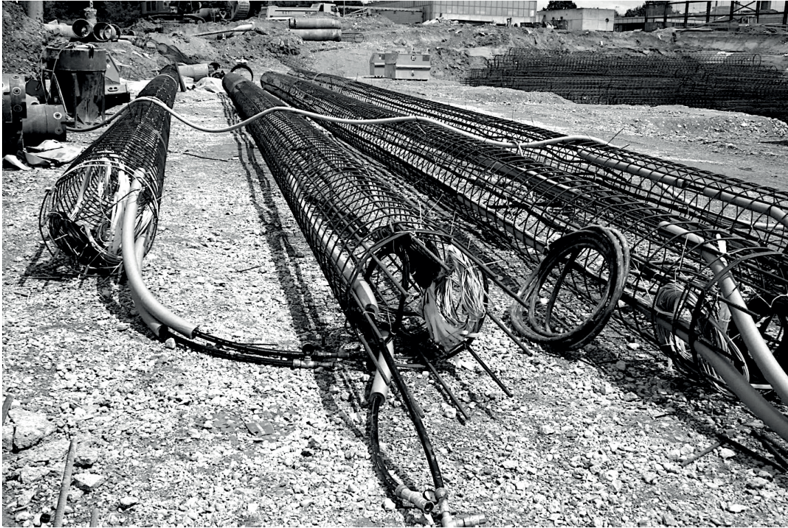
Figure 1.11: Examples of energy piles (image courtesy of Dr. Thomas Mimouni).
