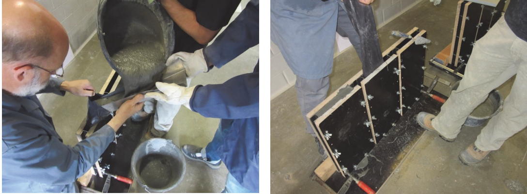
Figure 6-3. Specimen fabrication: (a) vertical casting of the fresh UHPFRC and (b) details of the forms.
