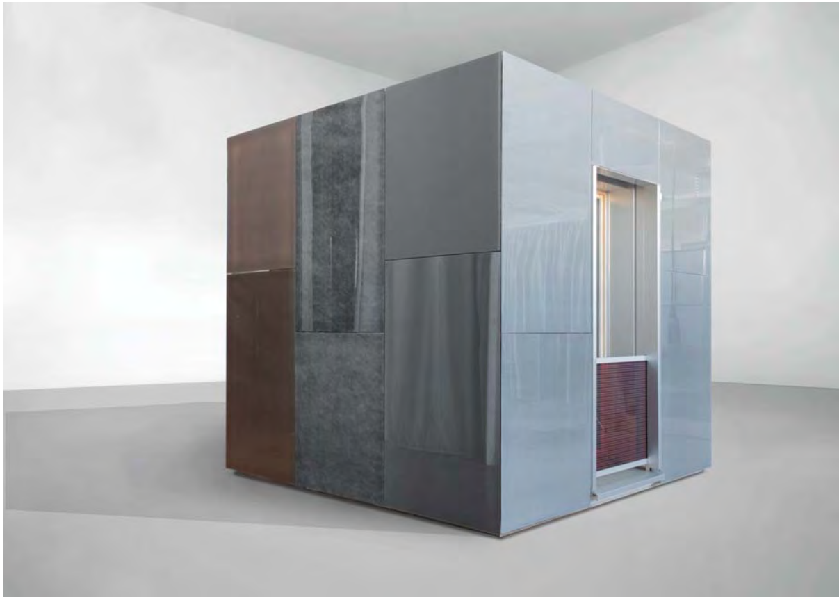
Figure 9. AAF full scale prototype. The prototype design allows to understand its composition and the way BIPV panels can be integrated in a low-carbon façade.
