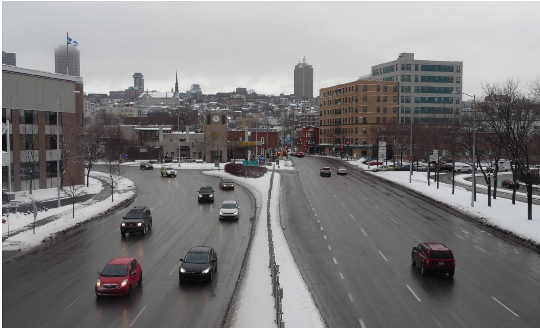
Figure 4:2 Photo of Quebec City seen from Autoroute Laurentienne 79
