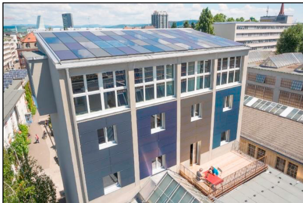
Fig. 5. The Kohlesilo in Basel. South façade with (from the left to the right) grey, blue, gold and green colour (11.3m 2 for each colours). The roof is a patchwork of black standard modules, grey, blue, gold and green coloured modules (total 81.7m 2 ). The north facade is not visible but represents 33.1m 2 .
