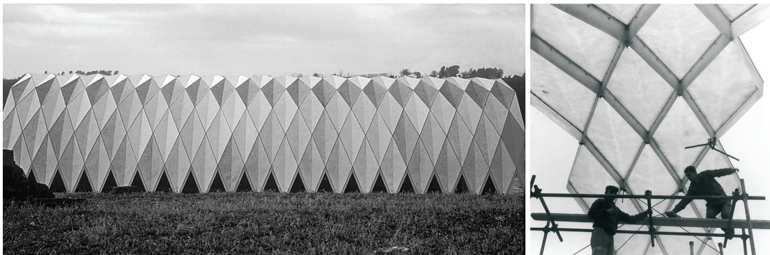
Figure 1.7 – Sulphur Extraction Factory by R. Piano, 1966. The thin folded sheets of reinforced polyester provide strength, stiffness and stability with minimum weight and also make the covered area very bright [67].
