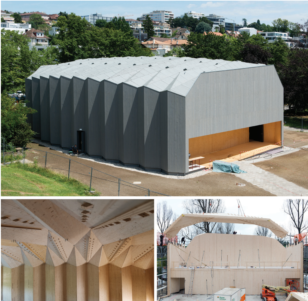
Figure 6.1 – Vidy Theater Pavilion, Lausanne, Switzerland [54]; (above) exterior view of the structure with a visible doubly curved form; (below left) the interior view with the featured closed slot MTSJ roof details; and (below right) the on-site assembly of the prefabricated roof segment.
