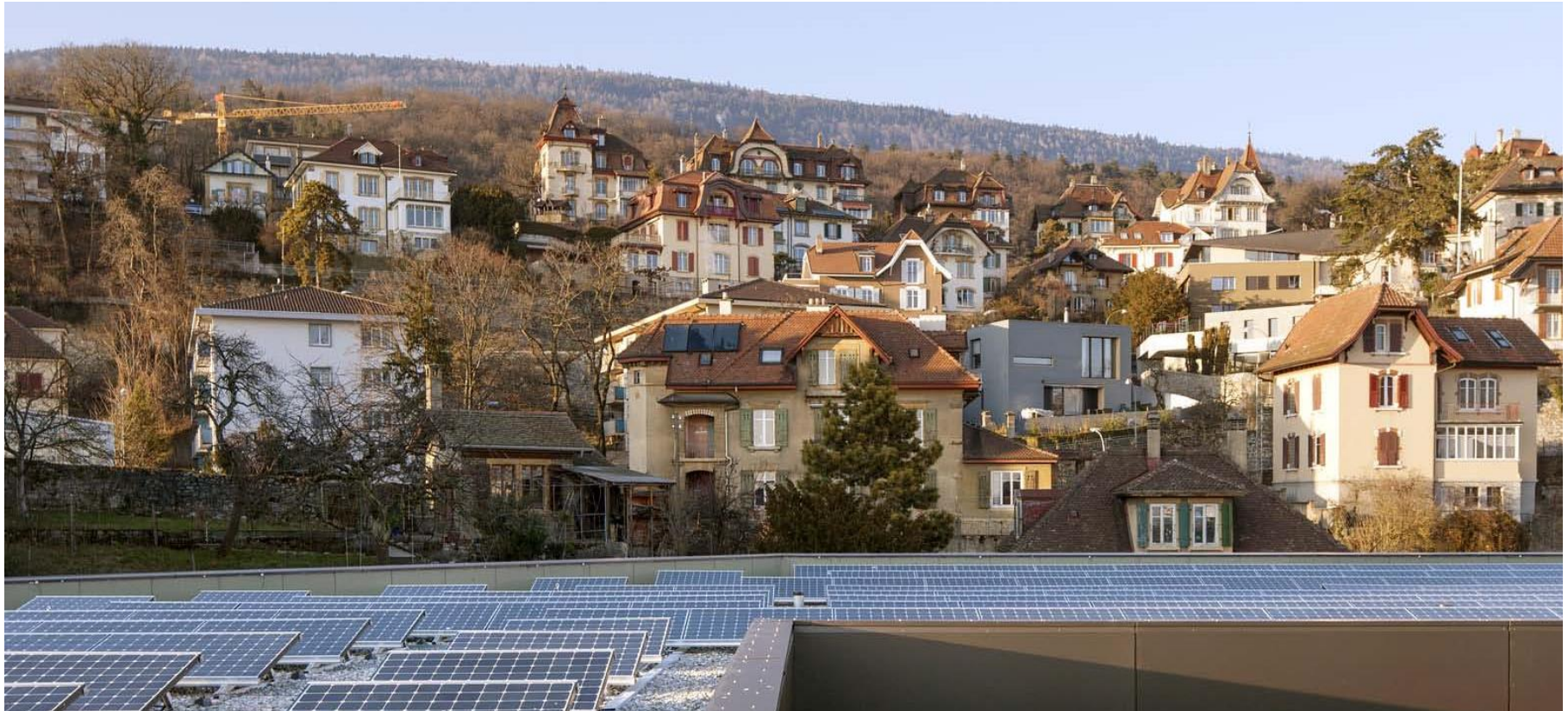
View from Microcity building roof | Neuchâtel
