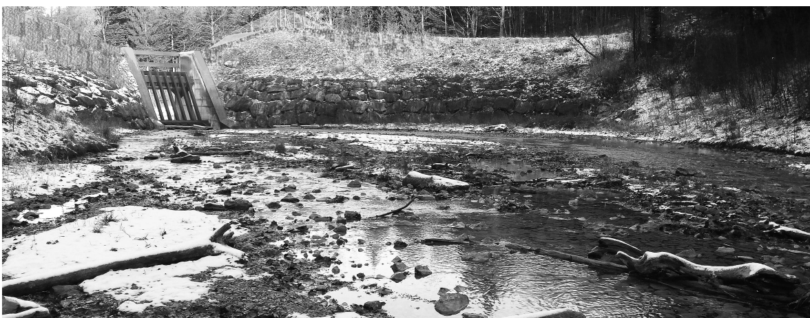
Figure 1.1 – A typical sediment trap with torrential barrier (left) for flow control, with upstream deposition area (Jenbach, Germany). © S. Schwindt.
