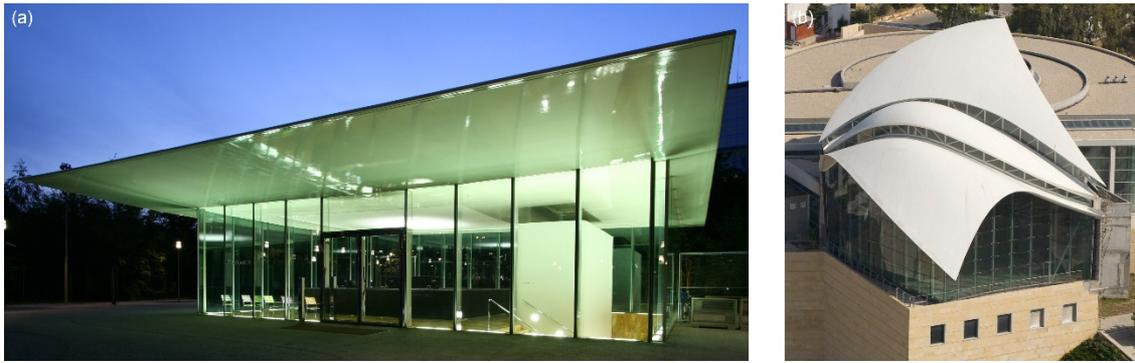
Figure 1.2 – (a) Novartis Campus Entrance Building: GFRP-PUR sandwich roof, Switzerland, 2006;<sup>2</sup> (b) Yitzhak Rabin Center: GFRP-polyurethane sandwich roof, Israel, 2006.
