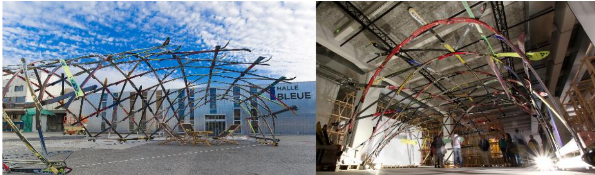
Figure 2. The ski pavilion: second assembly in the courtyard of the Blue Factory, Fribourg CH, on the left; fourth assembly in La Sucrière for the “Biennale Architecture Lyon” FR, June 2017, on the right. From left to right, three ballasts replace the connecting ropes and constrain the position of the three ground edges.
