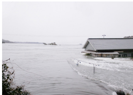
3. 15:25, March 11, 2011 Tsunami went beyond the seawall
