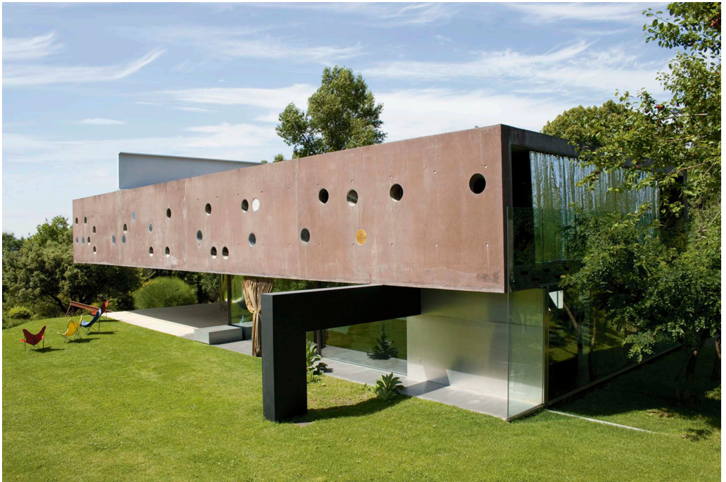
Exterior view of Villa Floirac , Hans Werlemann
