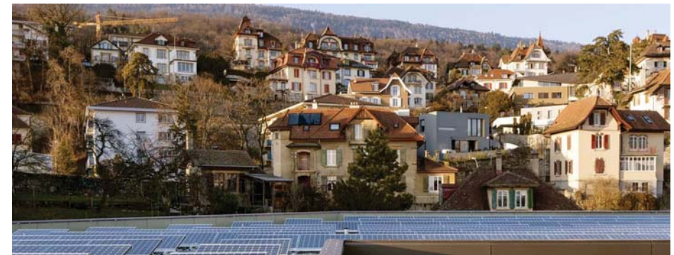
View from Microcity building roof | Neuchâtel
