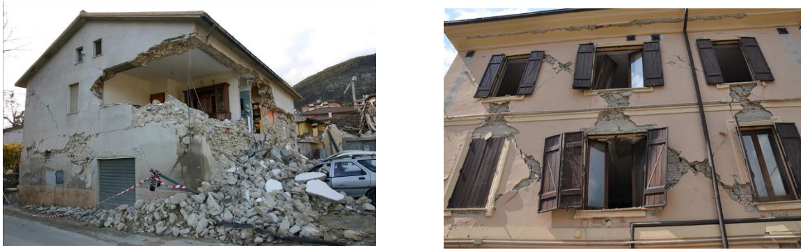
10 Fig. 1 Stone masonry buildings after the 2009 L'Aquila earthquake that failed due to an out-of-plane mechanism (a, Photo: 11 A. Dazio) and an in-plane mechanisms (b, Photo: A. Penna).
