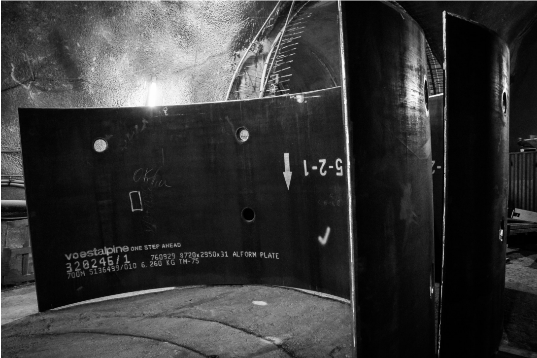
(a) Two rolled plates before welding and erection.
