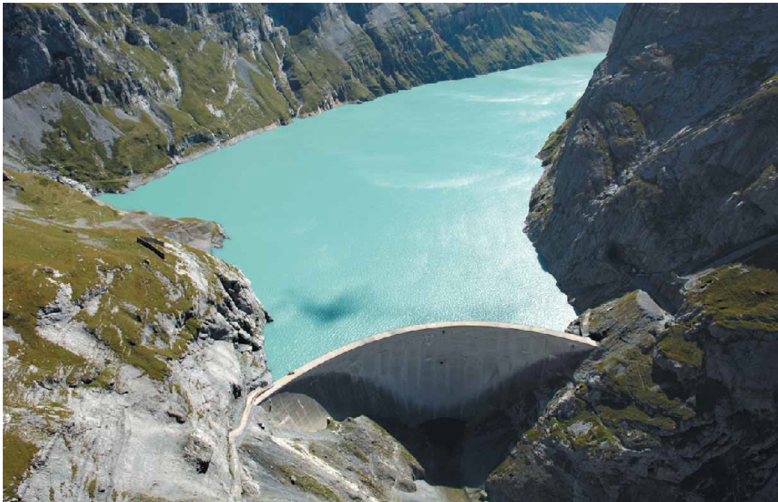
Figure 9.2: Photo of the Limmernboden dam (SwissCOD, 2011).
