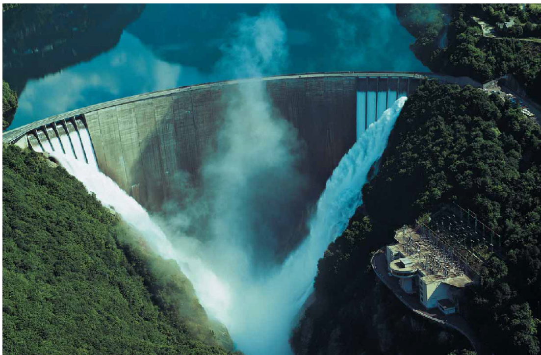
Figure 9.30: Photo of the Contra dam (SwissCOD, 2011).
