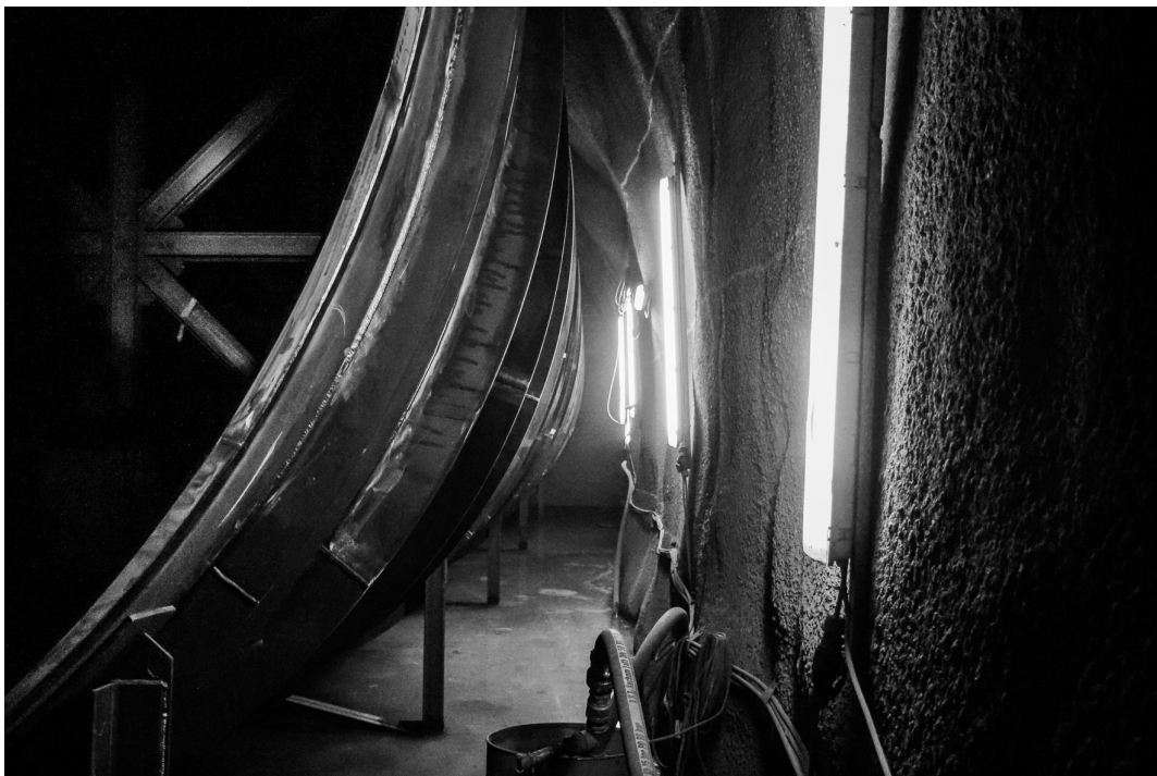
(f) Void between the steel liner and the surrounding rock (with shotcrete), before backfilling with concrete.
