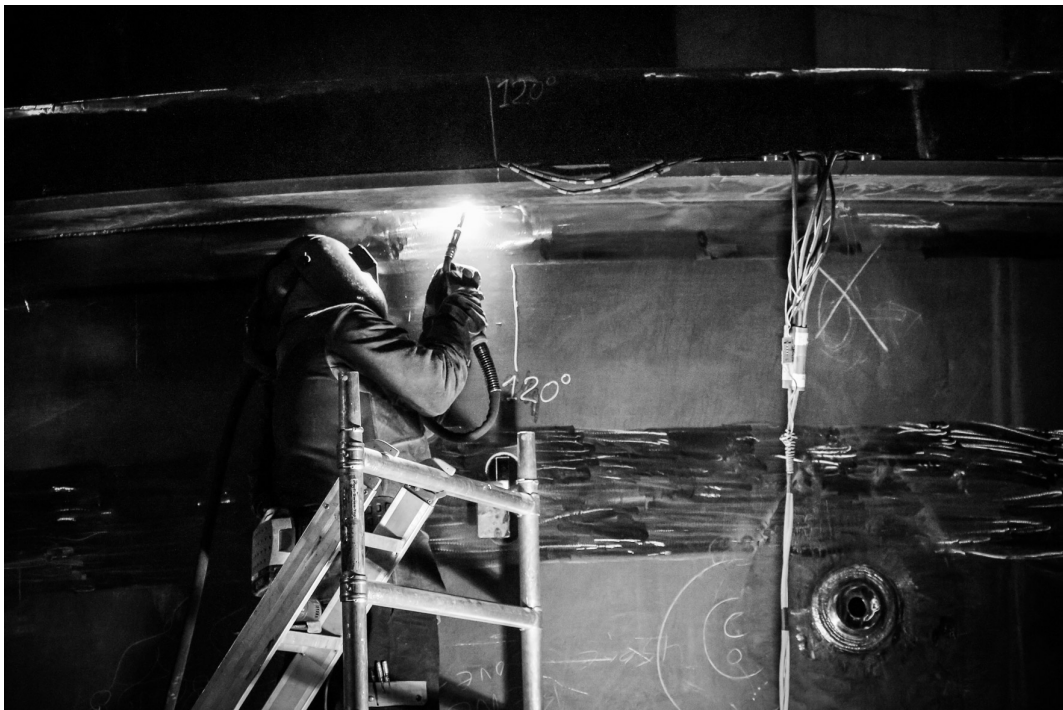
(b) Welding of an anchor ring.
