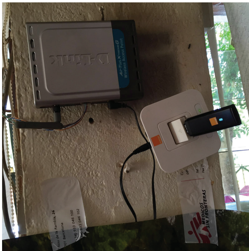
Figure 1.11 – A 3G mobile Internet stick mounted on the wall provides Internet access in the MSF mission in Kampala, Uganda.
