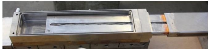
Fig. 5. The cable, in which the outer layer of Cu wires is replaced by two copper U-profiles, is being slid into the termination box.
