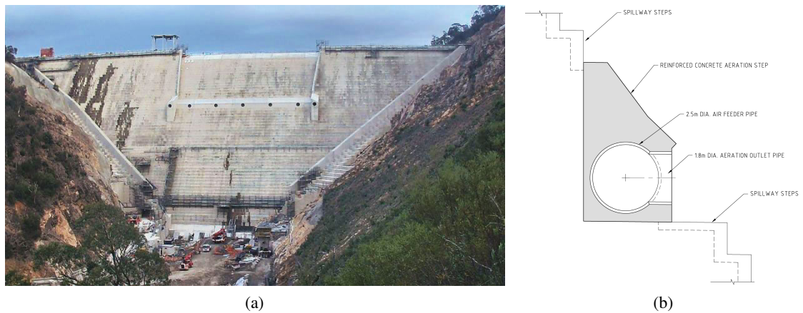
Figure 1.5 – Enlarged Cotter dam (a) construction photo (ACTEW, 2013), (b) aerator geometry (Willey et al. 2010)
