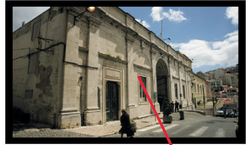
Hospital do Desterro, Colina de Santana (Intendente) (work in progress)
