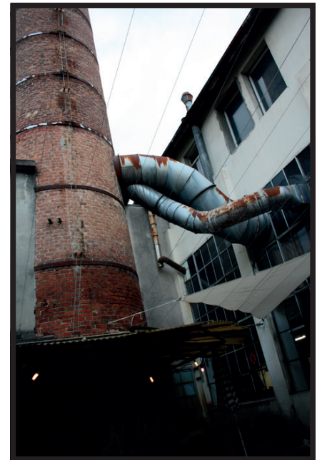
Img 334. traces of the industrial past (pipes and chimney).
