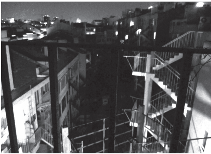
Img 107. The metallic staircase that connects the different floors and balconies of Prédio dos Anjos, leading to the roof terrace through the backyard patio.
