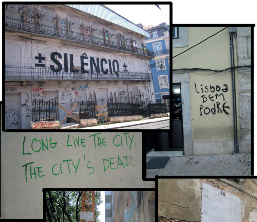
Img 55. The critique to the degraded material conditions of Lisbon's edifications (2012-13). >
