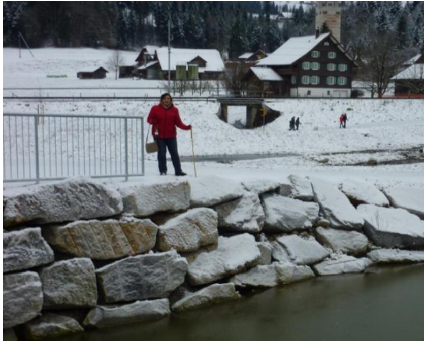
Figure 1.1 The view of large block size riprap and residential area in Switzerland (Kleine Emme 2011)
