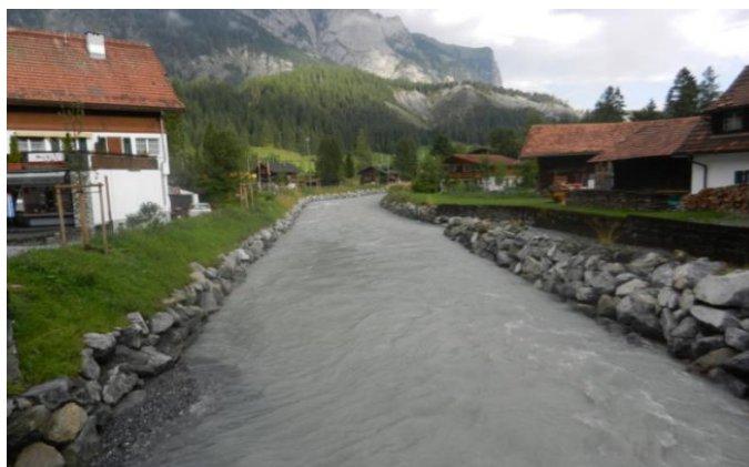
Figure 7.1 The view of riverbank riprap and residential area in the central part of Switzerland (Kander, Switzerland, 2012)
