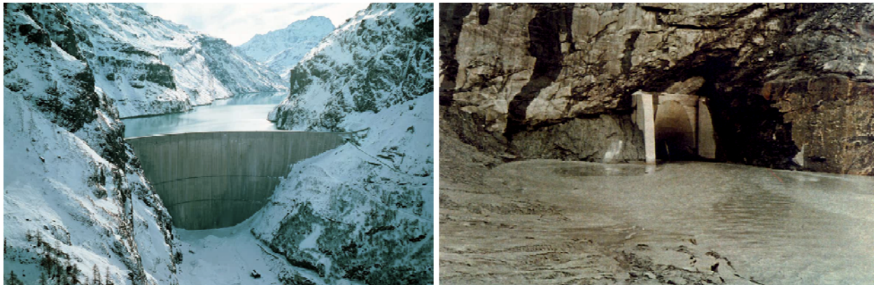
Fig. 1: (a) Mauvoisin dam (source: FMM) and (b) its bottom outlet showing high deposition
