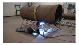
Figure 1.5 – The pipe welding machine in action during an indoor test. Guidance is provided by an expert, that closely monitors the welding torch while it turns around the pipe and manually adjusts the trajectory of the welding torch.
