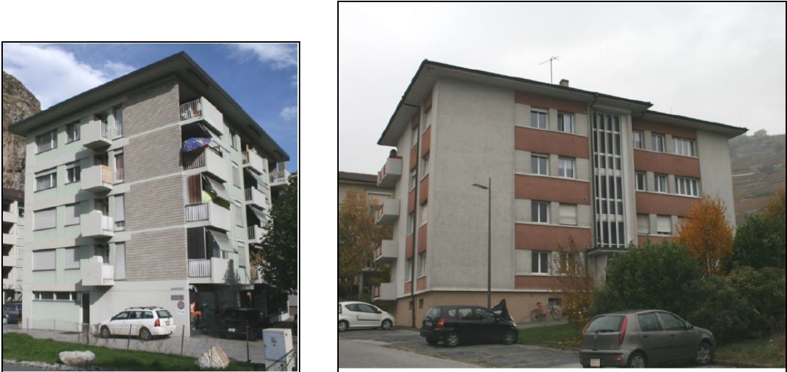
Figure 2 : Typical unreinforced masonry buildings in Switzerland.
