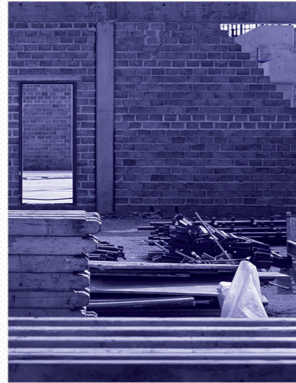
Fig. 3: Bricks and Beams : The shell of the airport's terminal building.
