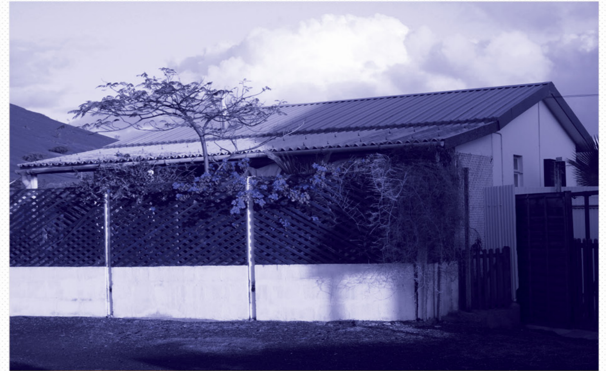
Fig. 37 : House and protecting vines
