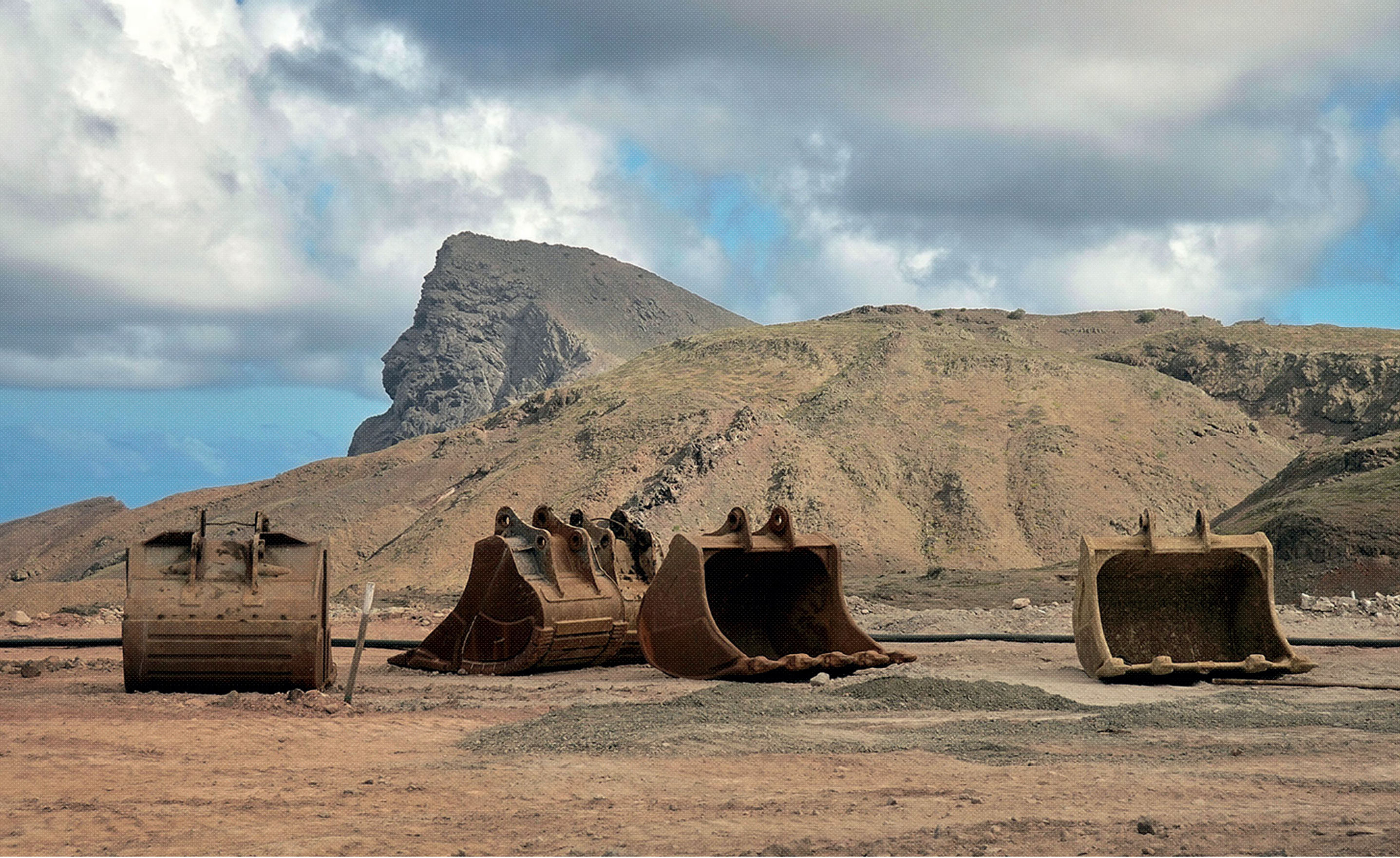
Fig. 16: Excavator buckets gather at the edge of the airport site. Austin Andrews, Frontier Empire I: Saint Helena . 2014
