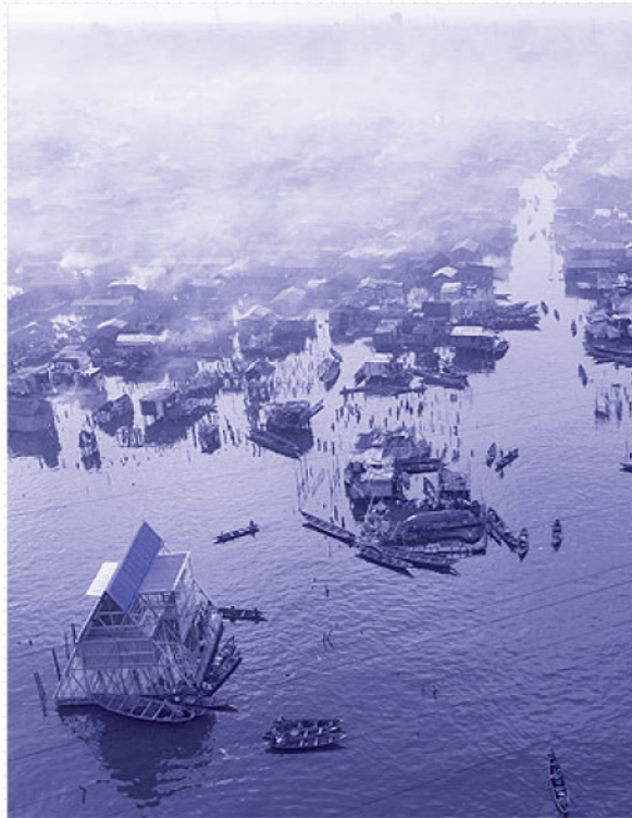
Fig. 8 : NLE Architecture, Floating school , Lagos, Nigeria, 2012 photograph by Iwan Baan
