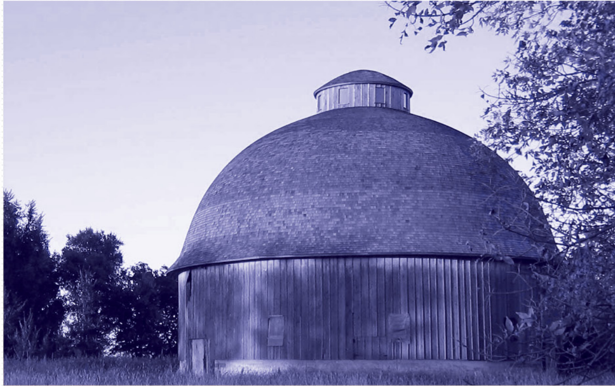
Fig. 22 : A round Barn that can still be found in the U.S. This example of round barn has a circular plan with on the top a natural ventilation system and sky-light openings.
