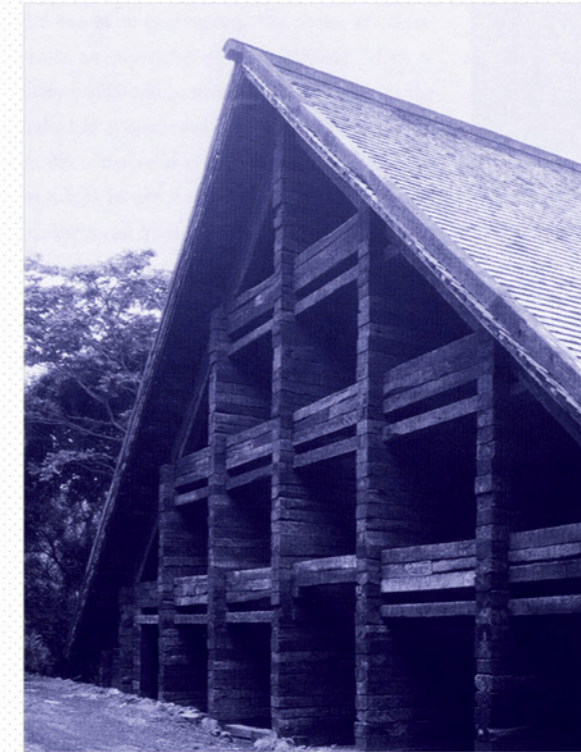
Fig. 10 : Shin Takasuga, Railway Sleeper house , Miyake Island, 1970' The house was built by using only old, wooden railway sleepers.
