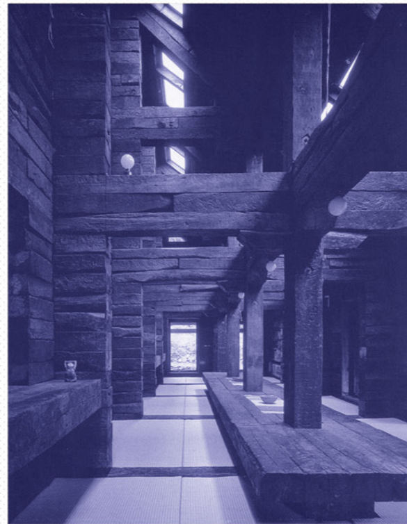
Fig. 24 : Shin Takasuga, Railway Sleeper house, Miyake Island, 1970' The house was built by using only old, wooden railway sleepers.
