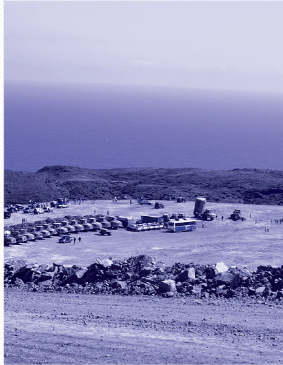
Fig. 9 : Saint Helena Airport construction.
