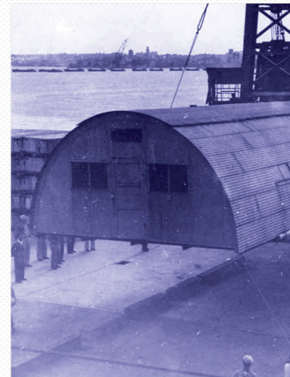
Fig. 18 : A Quonset hut being transported at the 598th Engineer Base Depot in Japan, post-World War II
