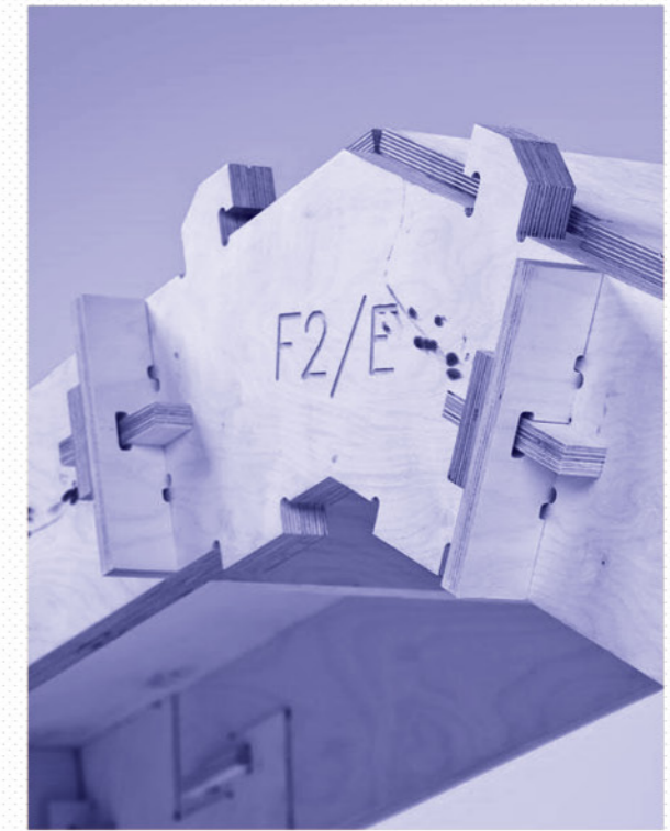
Details of a prefabricated wooden beams made from plywood panels. A new aesthetic is emerging.
