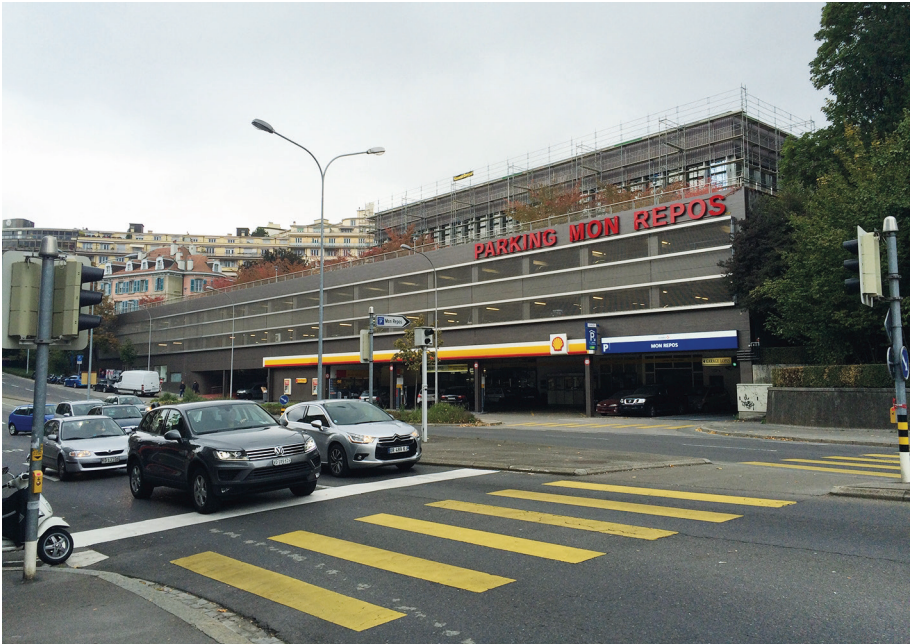
Parking-silo de Mon-Repos
