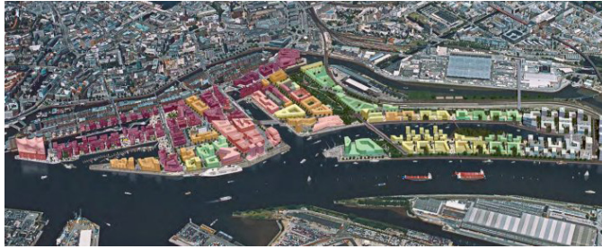
Hafencity, Hambourg, Michael Korol, 2014
