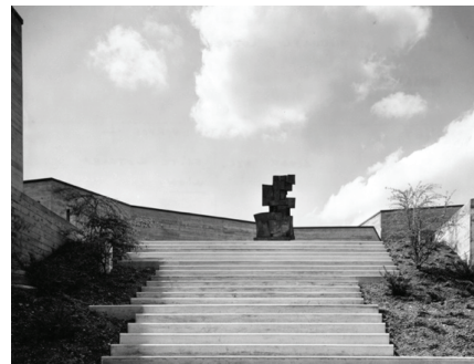
Figure 5.2-4: Before entering the courtyard, one has to climb up the wide and steep stairs. With permission for reuse from [203]
