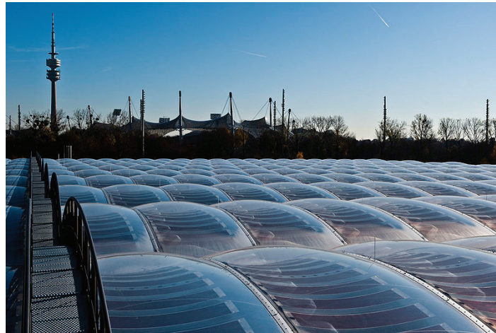
Figure 1.5-9: ETFE cushions roof with integrated photovoltaic cells of Munich's municipal waste management department by Ackermann & Partner (2011). (Photo credit: Michael Fischbacher)
