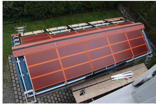
Figure 1.5-6: The coloured BIPV on a carport roof. Photo credit: Stephen Wittkopf.
