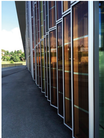
Figure 1.5-7: The Grätzel cells on the west facade of Swiss Convention Centre in EPFL.
