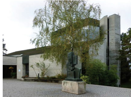
Figure 5.2-12. The main church building. Photo taken in 2012.
