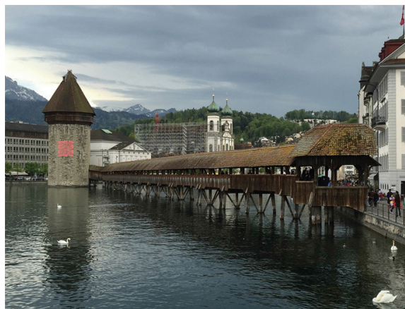
Figure 6.3-2: The Lucerne Watertower. The red area marks the location where BIPV are hypothetically placed.
