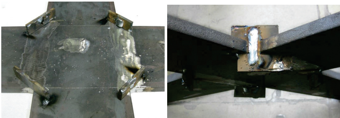
Figure 2.15 – Welds flush ground and sealing fillet welds done with auxiliary plates
