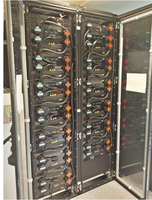
(b) Leclanché StoraXe® Storage Rack System SRS0029
