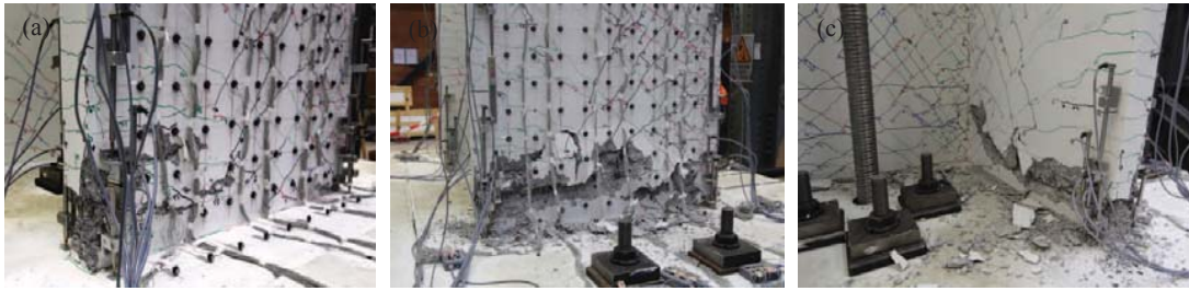
Figure 3.7: TUD: explosive compression failure of the distributed reinforcement layout flange (East flange). Wall condition at 1st cycle at position H at 1.5% drift (a-b) and wall condition after failure in the 2nd cycle at position H at 1.5% drift: view on the inner side (c) and view on the outer side (d).
