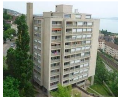
Figure 1: Building image (current status).
