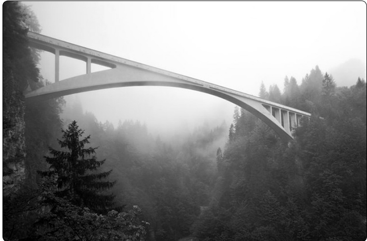
figure 2 the Salginatobel bridge designed by Robert Maillart, picture by Andrea Badrutt.
