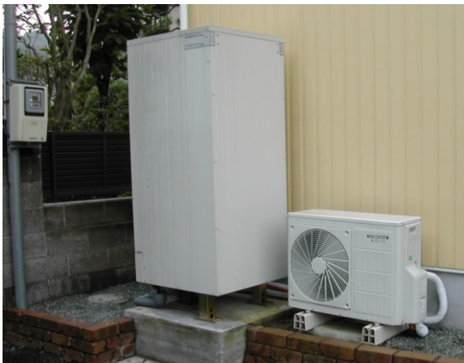
Figure 8. Eco Cute at my home. Heating capacity 6 kW, tank capacity 460 l, 2004 model.
