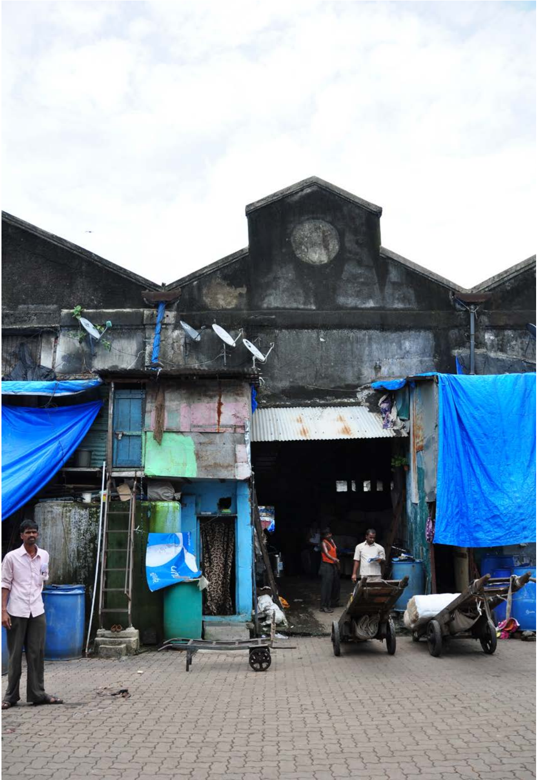
Warehouse entrance, Surat Street
