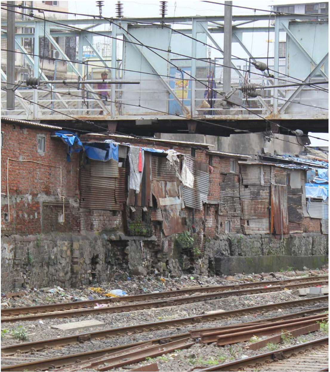
Dwellings built along railways, Masjid Bunder
