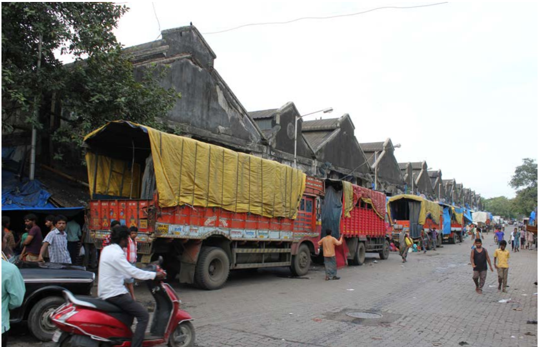
Trucks parked in front of warehouses, Yusuf Meher Ali Road
