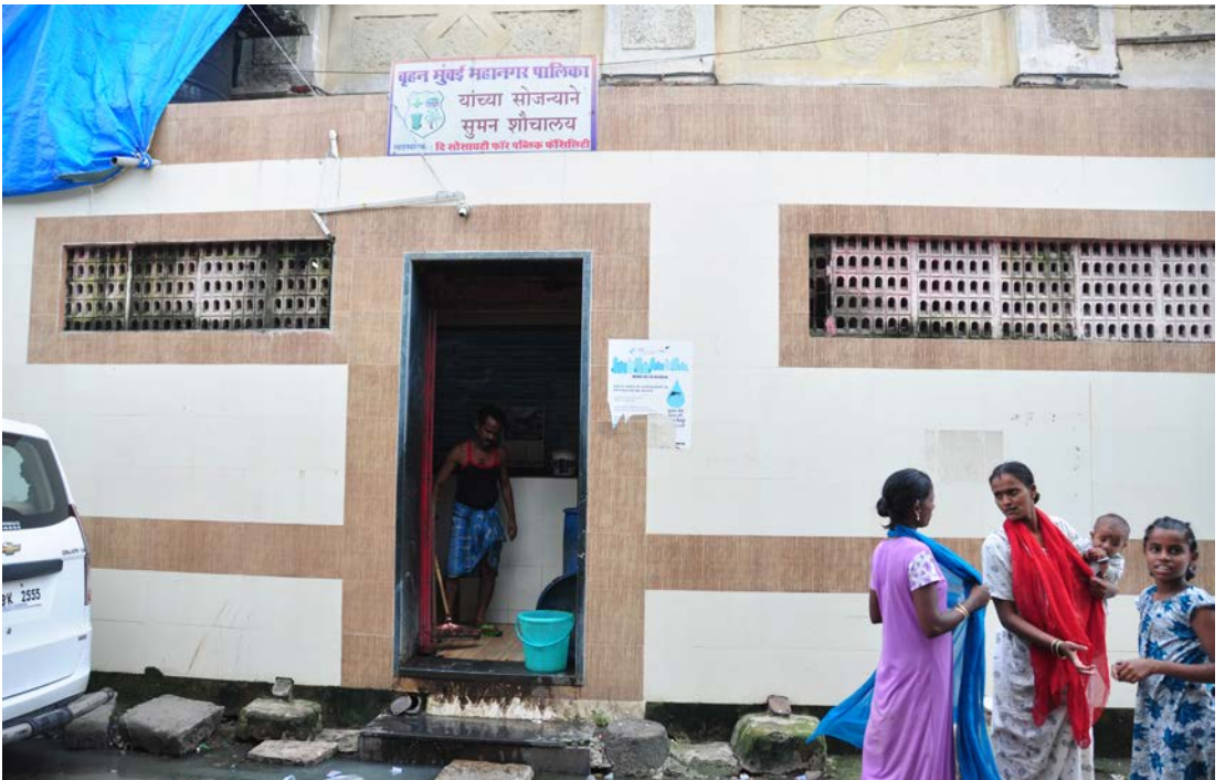
Government provided toilet blocks, Baburao Bobde Marg
