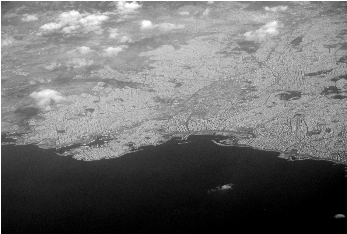
Aerial view of Piraeus and its port, the linear industrial axis including Pireos street and Eleonas and the centre of Athens
