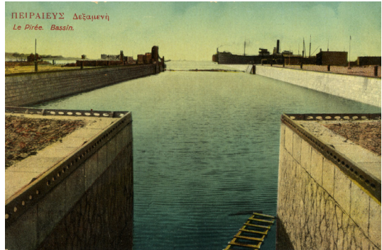
View of a basin
