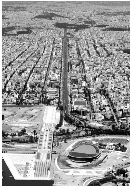
L. Syggrou linking the city centre with the waterfront
