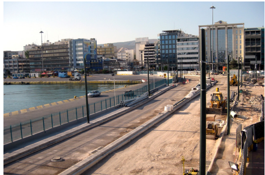
Fences around the port isolating it from the city
