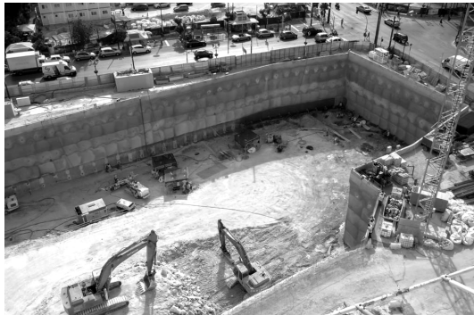
Dimotiko teatro station under construction in Piraeus
