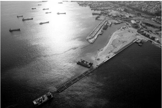
View of terminal III under construction
