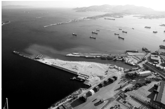
View of terminal III under construction
