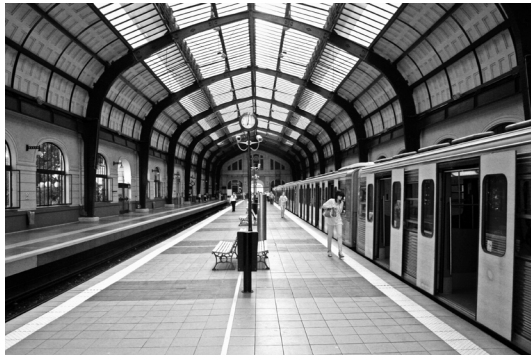
The above ground metro station of Piraeus
