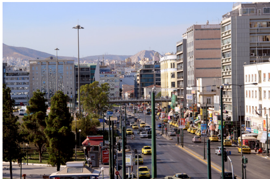
Piraeus port ring road and aerial bridge
