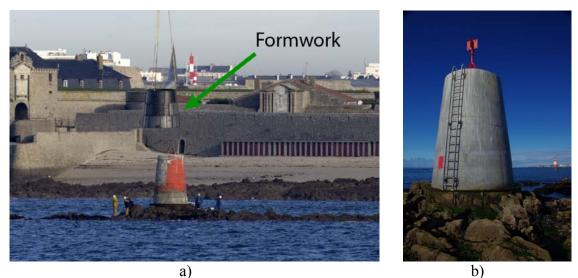
Figure 5: Application of UHPFRC, Cabon turret, Brittany, France, 4.2 m<sup>3</sup> UHPFRC applied by helicopter, 2013, a) installation of the formwork, b) finished UHPFRC surface.
