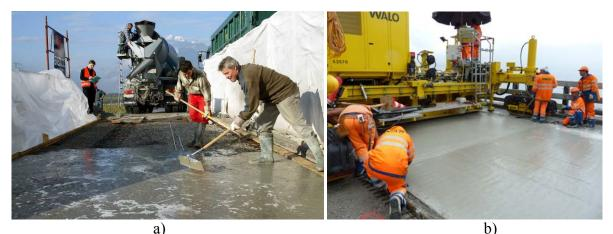
Figure 3: Application of UHPFRC. a) Bridge over river la Morge, Switzerland 6 m<sup>3</sup>, 2004, photo Alain Herzog, b) Chillon Viaduct, Switzerland–  $2 \times 1200 \text{ m}^3 - 2014/2015$ .
